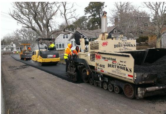
This year's Pavement Management Project (PMP) includes more than nine miles of street repairs. The majority of the work will consist of mill and overlays, with some spot curb repair.
