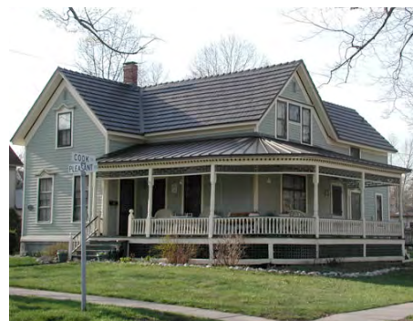
Metal shingles & standing seam roofing on a home
