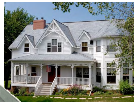
Recycled rubber roof shingles on a Iowa home
